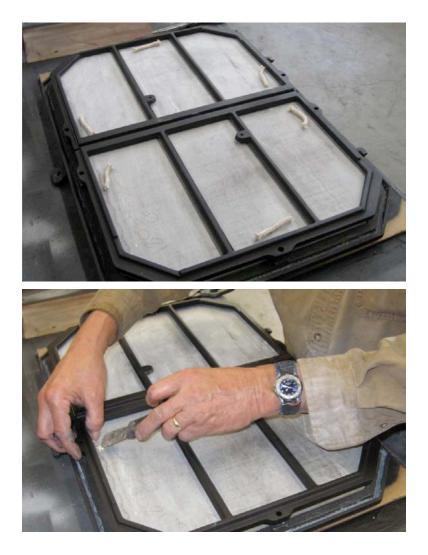
12. Tighten the screws evenly. Give each screw a few turns and repeat around the frame. Tighten the screws snugly, but do not over-tighten as this may lead to broken stone. With the screws completely tight you should be able to squeeze the retainer toward the lid and have no visible motion.
