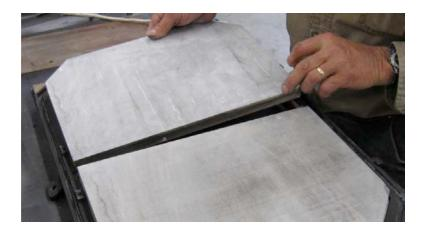
10. If the stone rests on the cast iron not the gasket, use a sander or flat file to remove stock from the edge of the two areas indicated in the following photo. Only remove enough to ensure a good fit (Maximum of 1/16")
